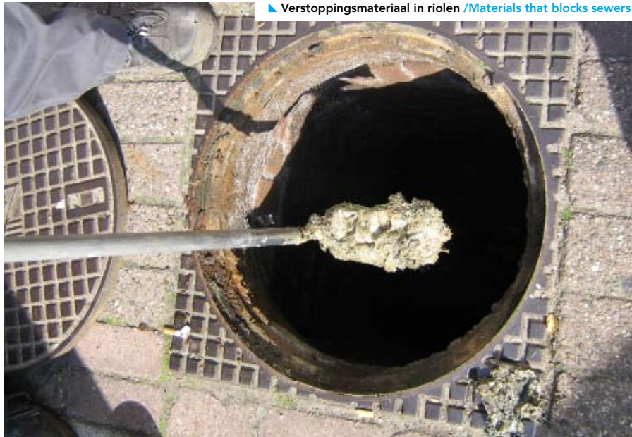
Verstoppingsmateriaal in riolen /Materials that blocks sewers
